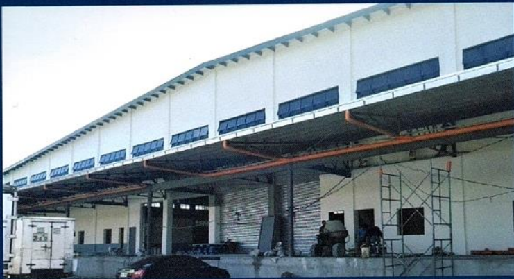
New 4-Bay Sucat Warehouse
