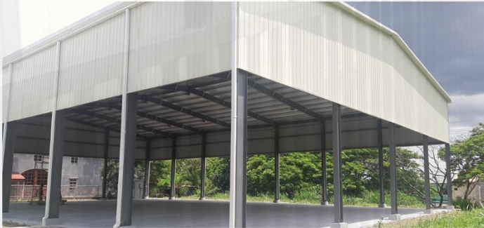
Community Basketball Court
